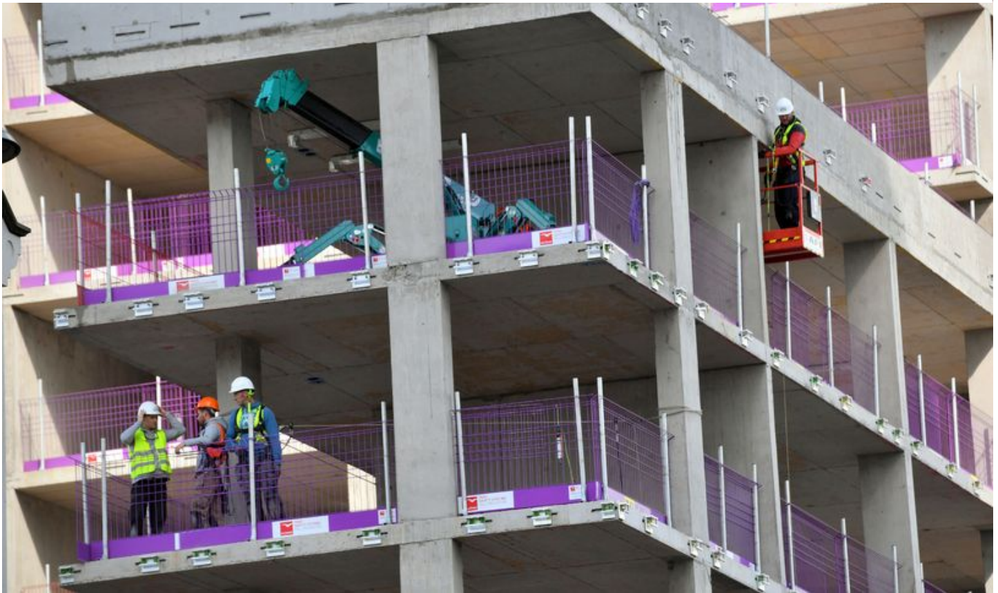
Student accommodation under construction in Cardiff (Image: Rob Browne)
